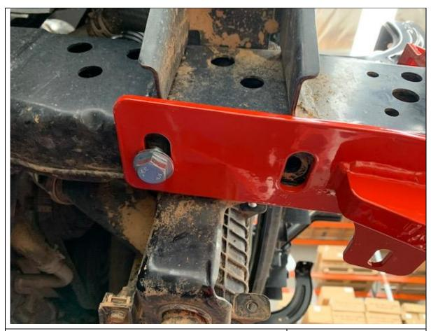
19. On Right hand side you will need to feed nut plates through to secure with M12x40 bolts
